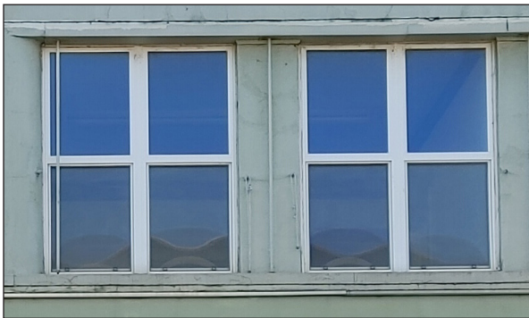
Figure 16: Metal Windows, 205 North Main St.
