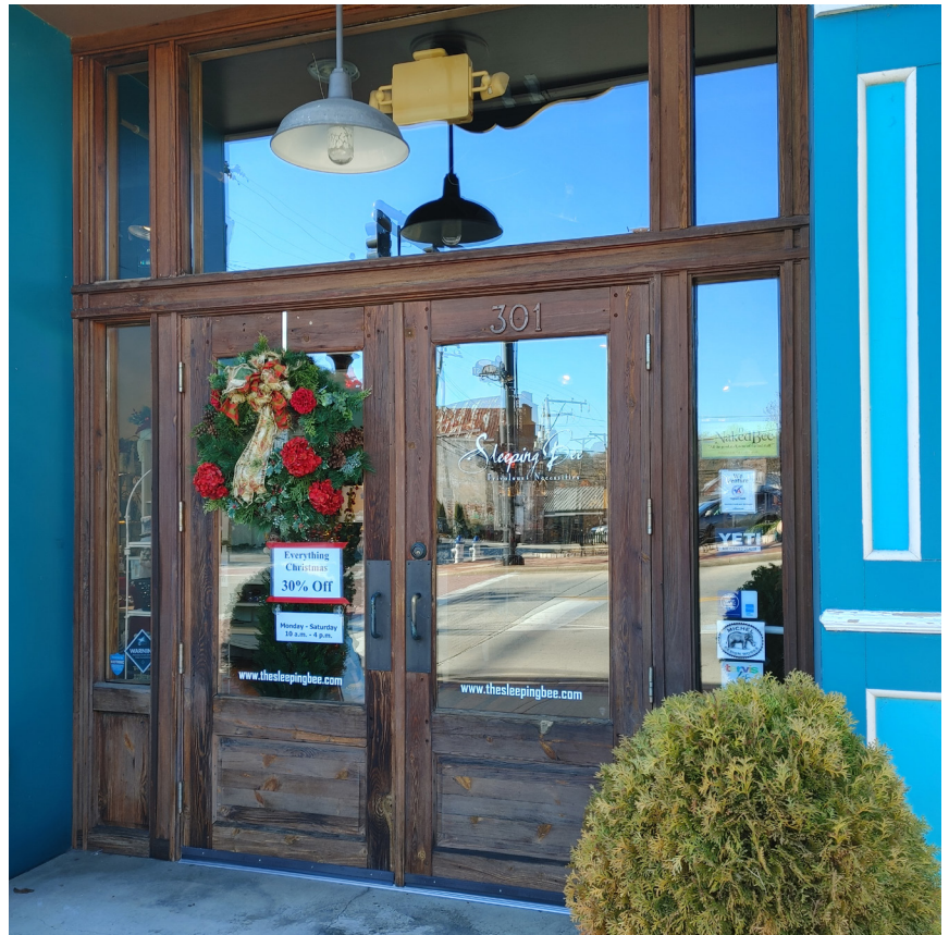
Figure 19: Double Wooden Door with side panels and transom.
